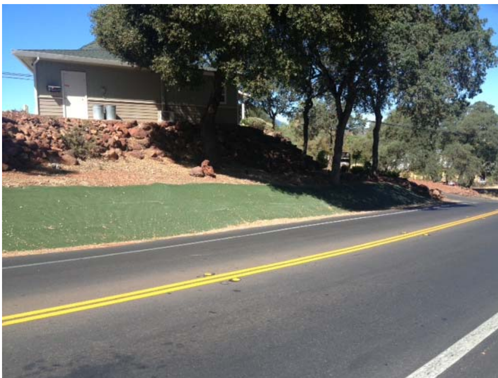
This photo shows an example of Post Construction BMP's that the City of Clearlake is requiring on construction projects. This erosion control blanket placed along a slope cut that was necessary to widen Old Hwy 53 south of Olympic Avenue to place class II bike lanes along Old Hwy 53.
